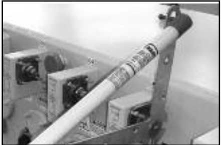
▲ Interrupter with dual operating handle.
