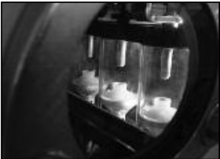
▲ Load break switch visible break.
