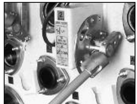
▲ Fault interrupter operating handle.
