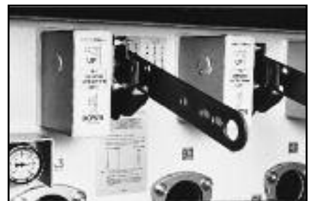
▲ Single phase interrupter operating handles.
