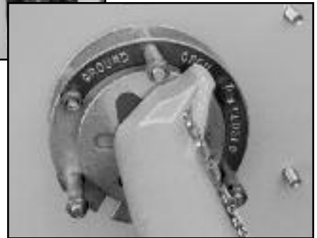
▲ Load break multi-position switch operator.
