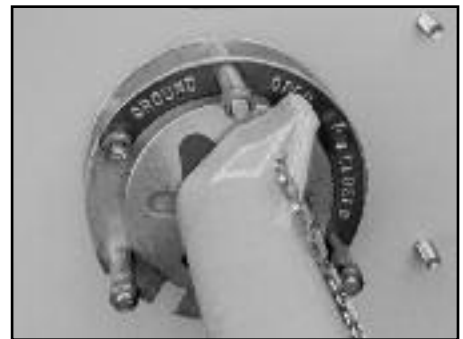
▲ Load break multi-position switch operator.
