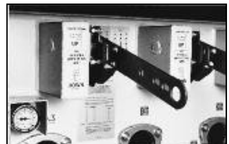
▲ Single phase interrupter operating handles.
