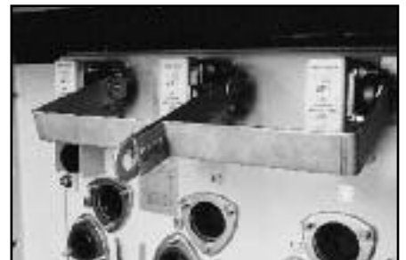
▲ Three phase interrupter operating handle.
