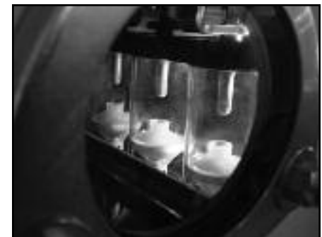
▲ Load break switch visible break.
