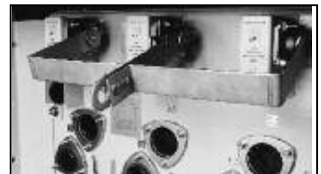
▲ Three phase interrupter operating handle.
