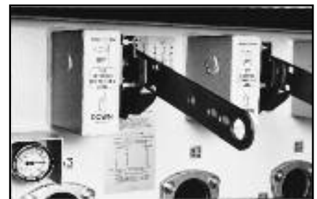
▲ Single phase interrupter operating handles.
