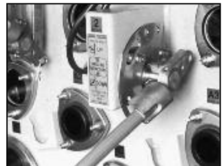
▲ Fault interrupter operating handle.
