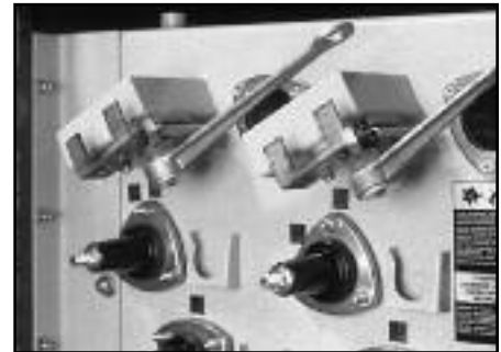
▲ Hookstick operable load break handle.
