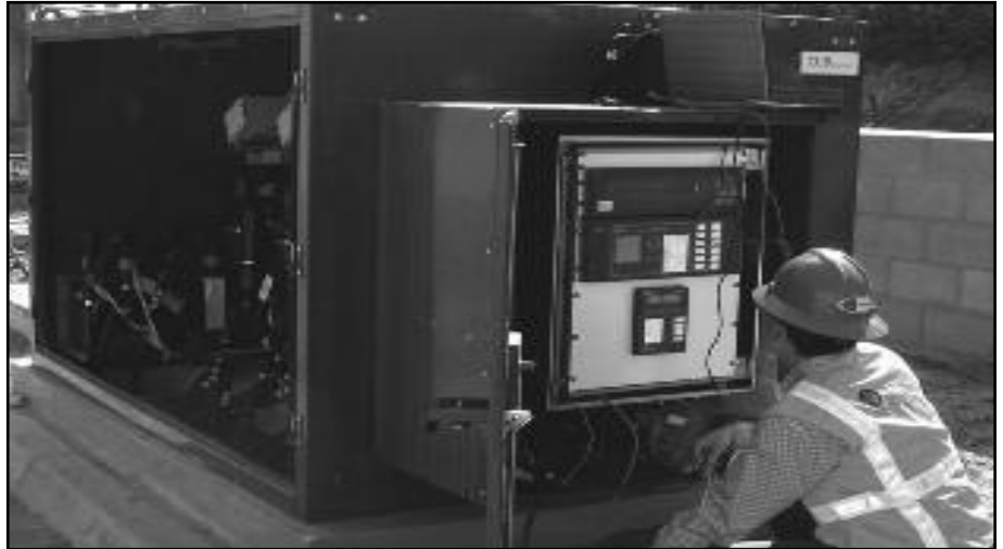
▲ Padmount switch with SEL controls.
