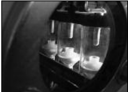
▲ Load break switch visible break.
