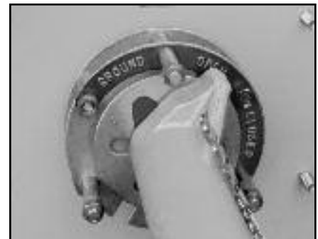
▲ Load break multi-position switch operator.
