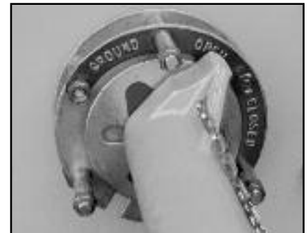
▲ Load break multi-position switch operator.
