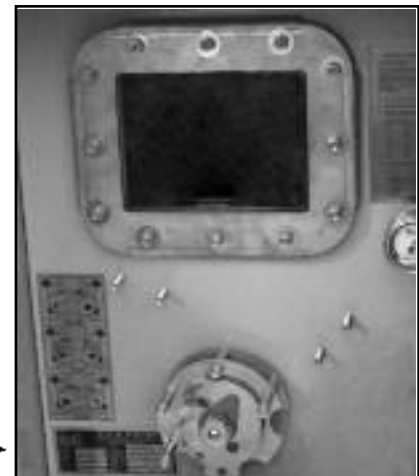
▲ Load break multi-position switch operator.
