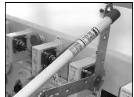
▲ Interrupter with dual operating handle.
