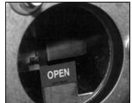
▲ Fault interrupter position indicator.
